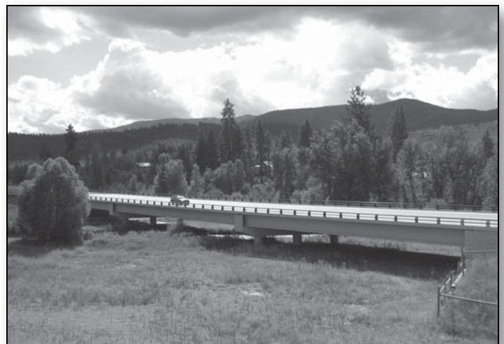
The new U.S. 93 multi-span Jocko River Bridge as it now crosses the Jocko River. The old highway consisted of a single span bridge, and long fill berms that constricted water and wildlife movement.
